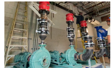
Pizzo K-8 School $3.5 Million - A/C Overhaul, Elevator, Fire Alarm System & Generator
