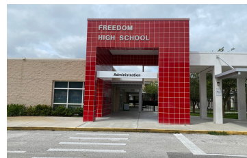
Freedom High School $6 Million - Partial A/C Overhaul, Fire Alarm System, Network Infrastructure
